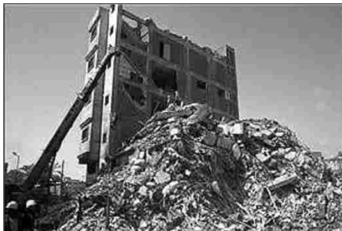
Figure 1-3 Collapse of clothing factory in Alexandria, Egypt ( Factory fire kills 15 in egypt.2000 )
