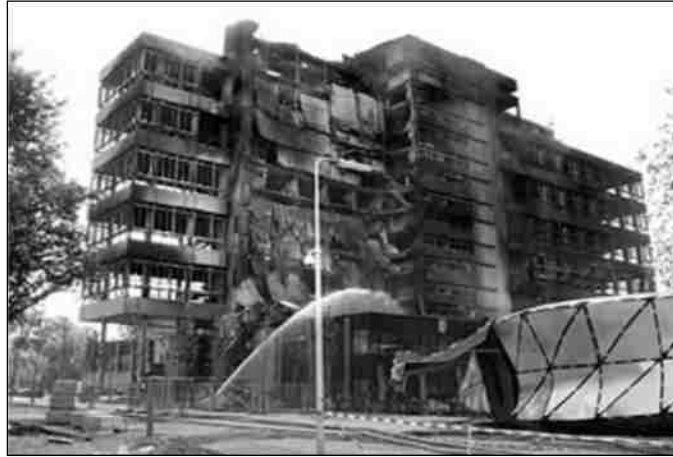
Figure 1-1 Collapse of Faculty of Architecture Building (Meacham et al., 2009)
