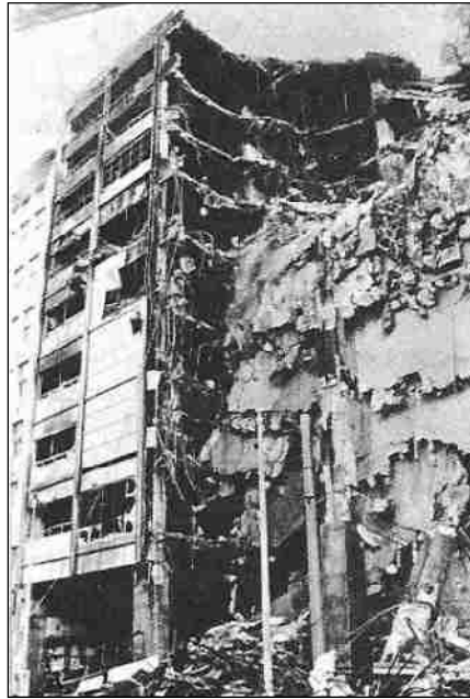
Figure 1-4 Collapse of Katrantzos Sports Department Store (Papaioannou, 1986)
